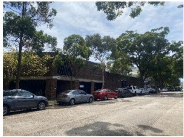
View looking north-west on Young Street along frontage of site taken from eastern side of Young Street.
